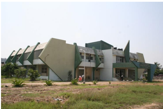
ANIMAL HOUSE FACILITY BUILDING TARAMANI CAMPUS
